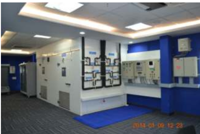
Live Freezer/Chiller Rooms
