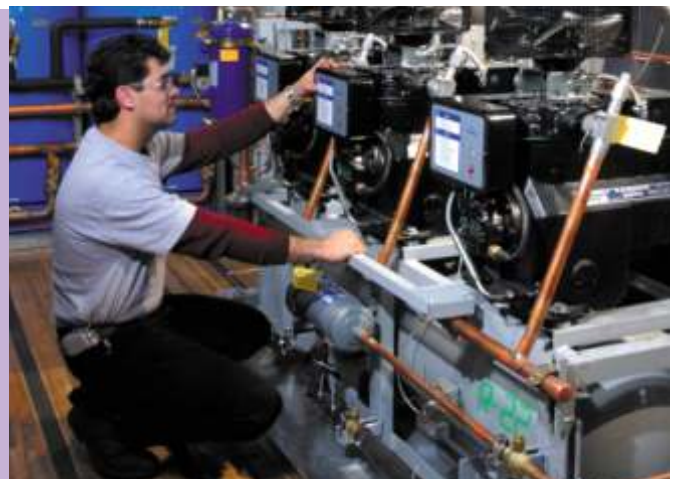
Advanced Refrigeration Controls/Remote Monitoring Systems
