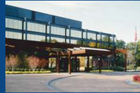
Headquarters in St. Louis, Mo.
